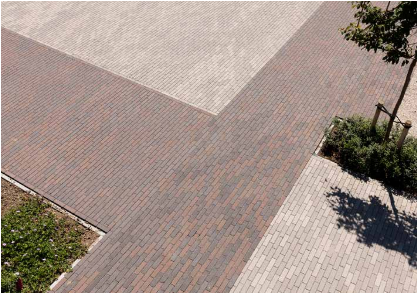
AQUATA BROWN Dudzele Village Centre, Belgium
