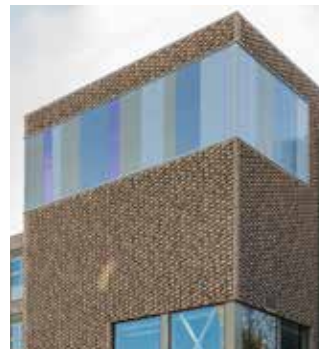
Paxton Primary School, Lambeth, UK Corium 50mm projecting tiles
