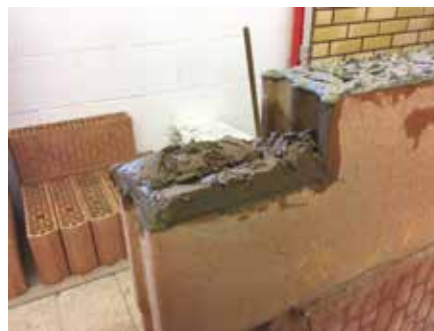
2. The lintels are installed using traditional mortar on the bearings.
