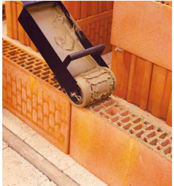
2. Roll the blocks on the floor or across the top of the pallet.
