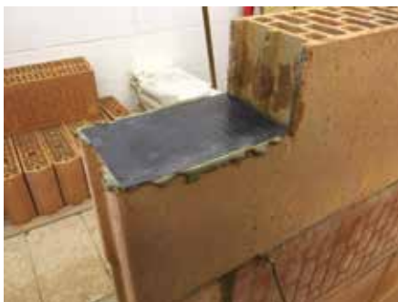
1. A piece of DPC should be laid on the bearings using Zero Plus mortar.
