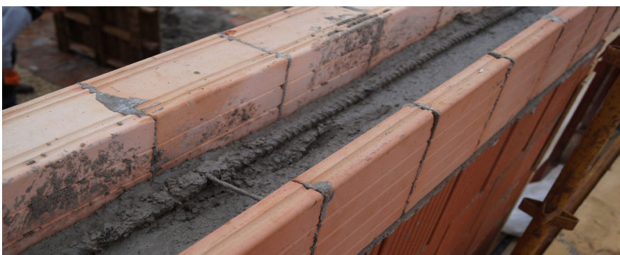
U SCHALE FILLED WITH CONCRETE
