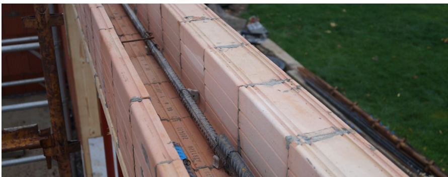
REINFORCING STEEL LAID INTO CHANNEL
