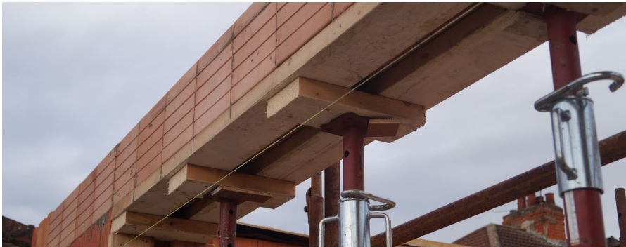
U SCHALE LAID IN POSITION ON TEMPORARY TIMBER SUPPORT
