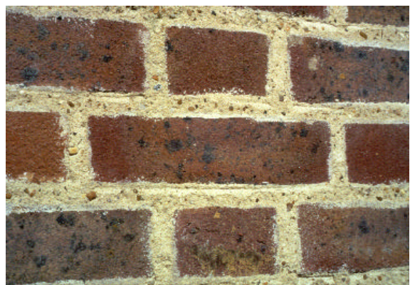
Characteristic appearance of Hydraulic Lime Mortar
