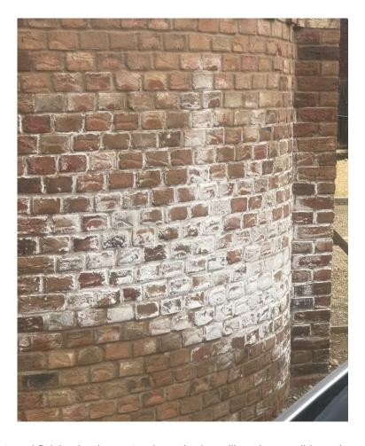
Should efflorescence occur where brickwork is the natural internal finish, clearly a natural weathering will not be possible and a spray application should be avoided. The appearnce of internall brickwork can be improved by applying a damp sponge, rinsed frequently in clean water, to encourage soluble salts to transfer to the sponge. it may be necessary to repeat the treatment.
